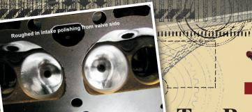
Roughed in intake polishing from port side
